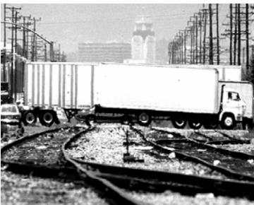
Before: truck crosses tracks prior to building Corridor.
